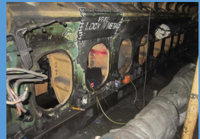
As Completed Repair of Crankcase Window
