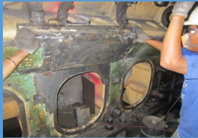
Replacement Casting In Place and Metal stitched
